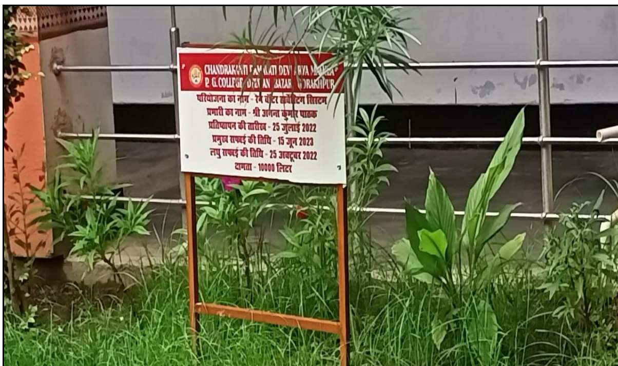
Fig.3.3 Rainwater harvesting system
