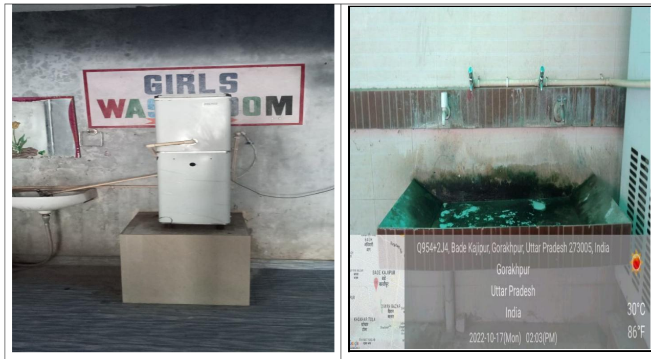
Fig. 2.3 Water Cooler and taps
