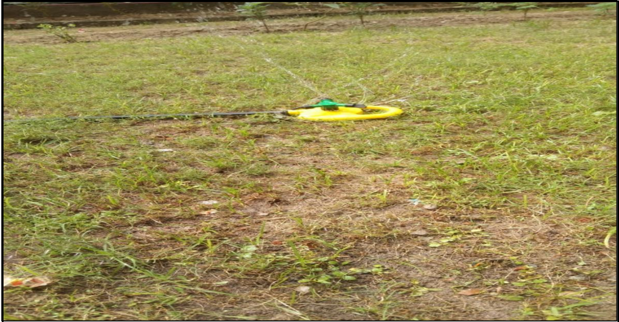
Fig.2.4 Water Sprinkler system in college campus
