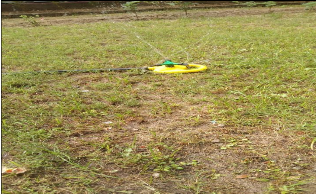
Figure:-Water Sprinkler system in college campus
